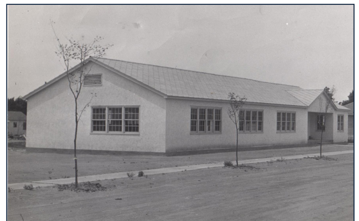
The parish hall is made of a former officers' barracks, halved and joined at right angles. Stuccoed on the outside, the hall is finished on the interior in knotty pine. At present time the hall is being used for catechetical instructions.
